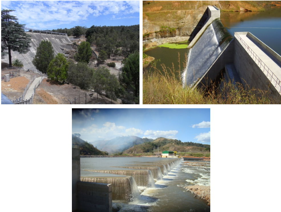
Fig. 1. Illustration of dam structures: a) Traditional smooth chute, b) Flow over a stepped chute, c) Labyrinth (Picture acknowledgements: Fig.1a: Stuart Longley; Fig.1b and Fig.1c: Engevix Company).
